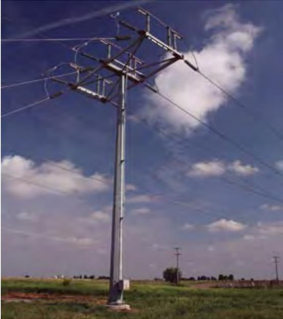
ROHN can optimize pole designs based on customer requirements, manufacturing efficiencies and material availability. Preliminary calculation packages are sent to our customers for review and approval prior to manufacturing. Fabrication and erection drawings are produced in AutoCAD and accompany the structures we produce. Our commitment to the utility industry is to provide the highest quality products with the shortest lead time.
